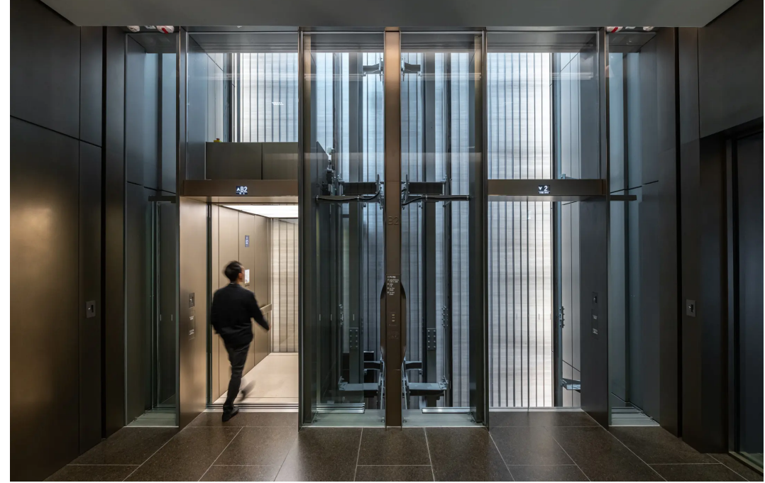
Glass elevators connect the lobby to the basement
